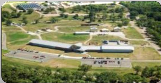
1LT Terry CBRN Responder Training Facility
