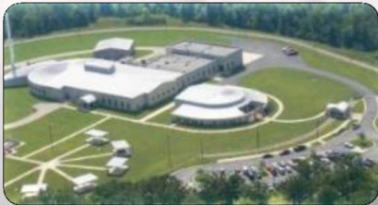
Chemical Defense Training Facility
